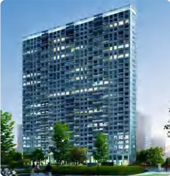
Office Building Machine Rooms
