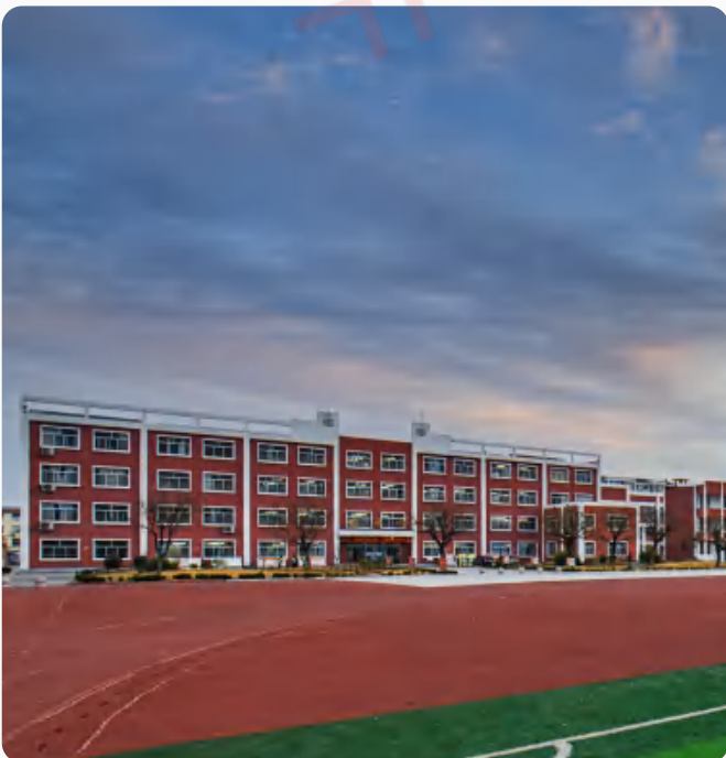
School Machine Rooms
